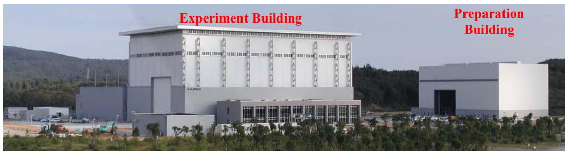
Photo 1 General view of E-Defense
